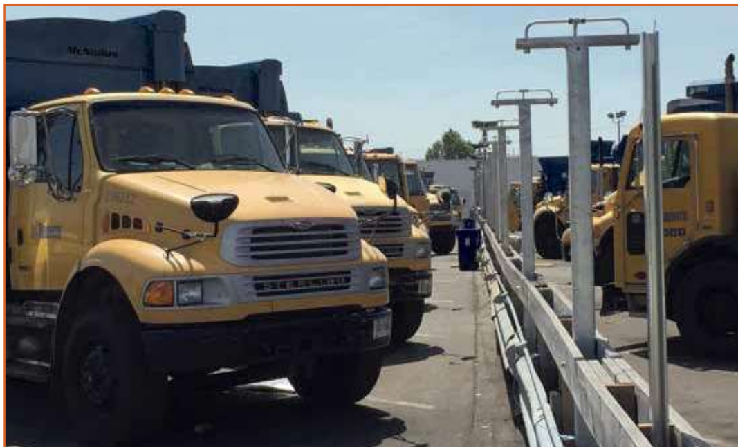
City of Toronto CNG fueling station
